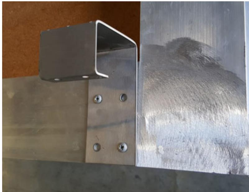
Note the edge of the cable clamp bracket lines up with the inside edge of the side rail and the bottom of the cable clamp bracket is level with the bottom rail of the gate.
