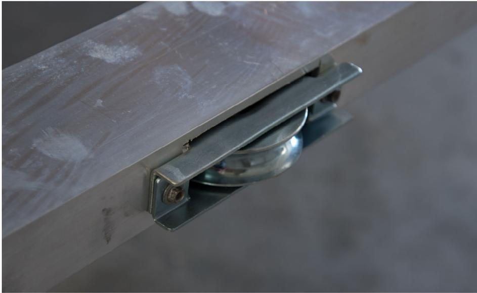
Make sure you are working with the outside face of the gate. This face will be to the outside and does not have your guide channel. Mark and drill a hole if not already done for your pulleys at each end. This hole is to be 50mm up from the bottom of the gate and 50mm in from each end.
