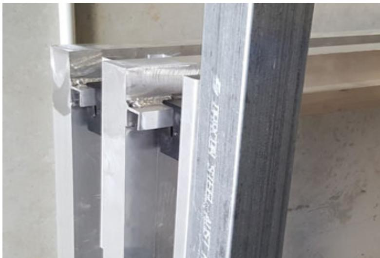
8. With both gates aligned the cable clamp bracket is now in position and by ensuring the cable is sitting in the inside corner of the bracket use the two Phillips Head Machine Screw to secure the cable at this point.
